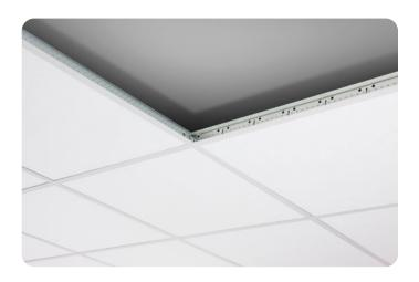
Parafon Decibel Light has a core of non-combustible stone wool and an aluminium membrane at the back and satisfies the lower requirements on sound insulation via the suspended ceiling. In combination with Parafon Decibel Barrier installed vertically in the plenum, or the sound absorbing Parafon Bass placed on top of the suspended ceiling, the sound insulation with Decibel Light can be reinforced significantly if required.
