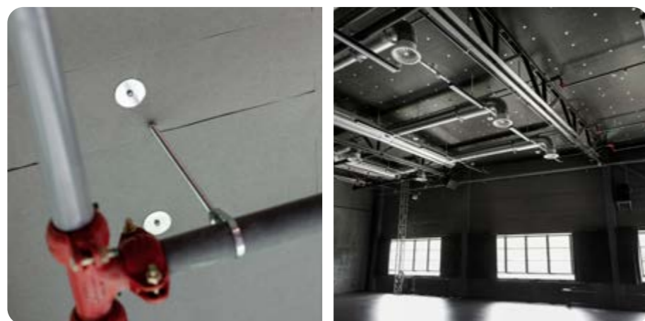
PRODUCTS: PARAFON BULLER, 50 MM GREY AND BLACK INSTALLATION: DIRECT MOUNTING WITH WASHER AND SCREW.
