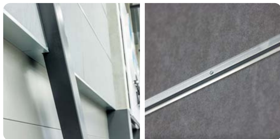
THE ABSORBERS ON THE ARENA'S SHORT WALLS ARE MOUNTED WITH MT PROFILES LEAVING SPACE BEHIND THE PANELS.
