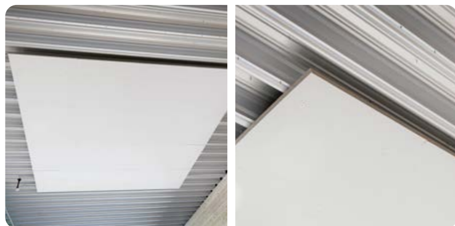
PARAFON BULLER TILES MOUNTED ONLY PARTIALLY COVERING THE CEILING WHICH MAKES THE INSTALLATION FASTER AND EASIER.
